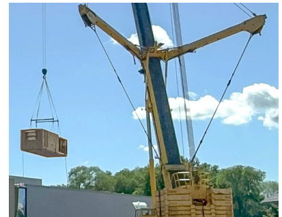
Crane installation of this one-section XeteX RTU.
