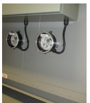
Bipolar ionization system
